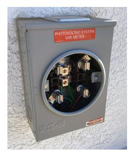
Meter sockets must be covered with an approved meter socket cover. Do not leave a meter socket exposed or use conductive materials as a cover.
